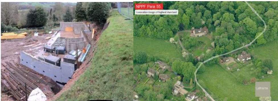
Figure 1: (a) Aerial view of the site location; and (b) Site build progress.
