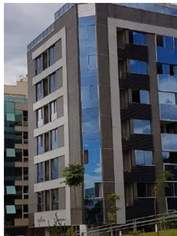
Figure 3: Building C (dark colour used).
