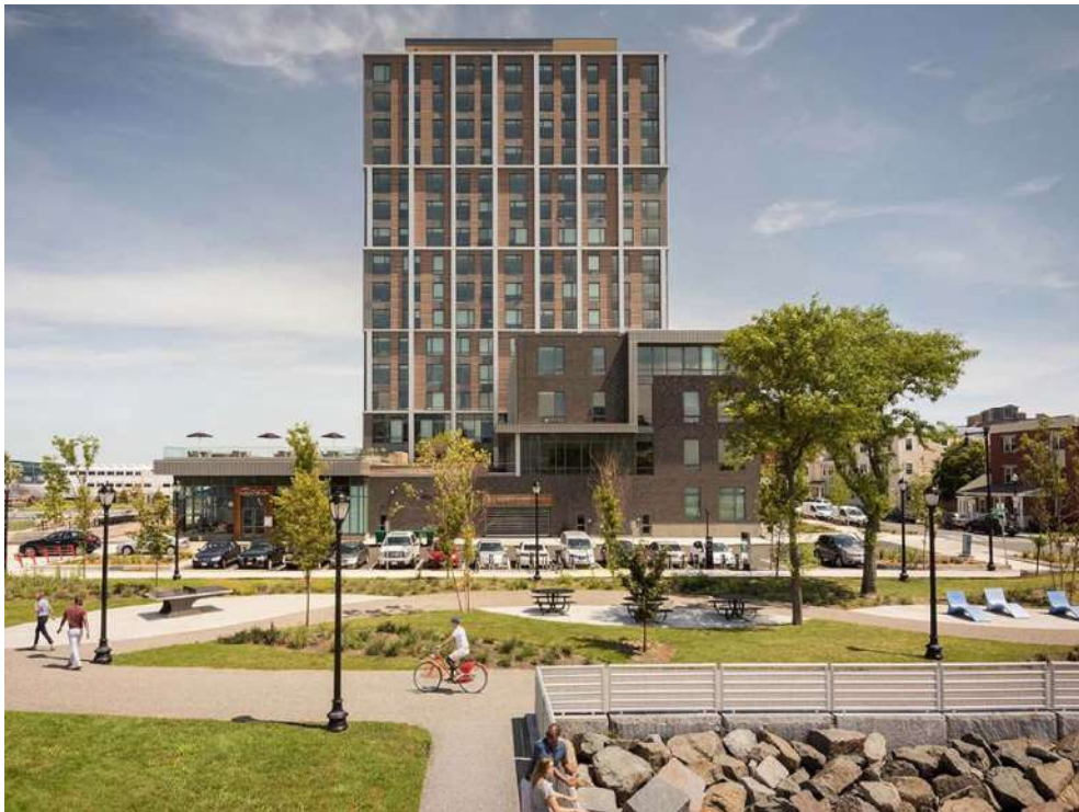
Figure 7: The enhanced Harbor walk serves to protect the development via enhanced seawall and absorptive green spaces flanking the structure, which channel runoff and reduce storm surge force impacts. (Source: Stantec Buildings Group.)
