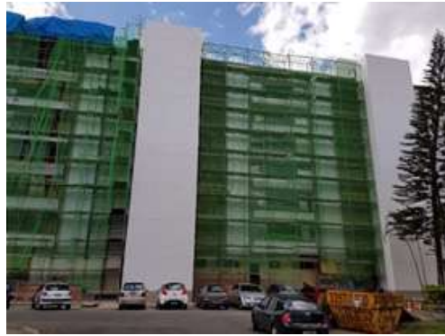
Figure 1: Building A (light colour tile used).
