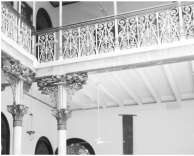
Figure 6: Victorian Scottish cast-iron columns and railings.
