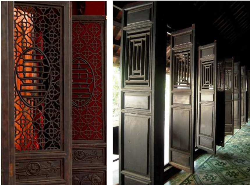
Figure 1: Left: Decorative lattice screens as means of passive ventilation and light control. Right: rotatable door panels with traditional patterns. ( Source: Author. )
