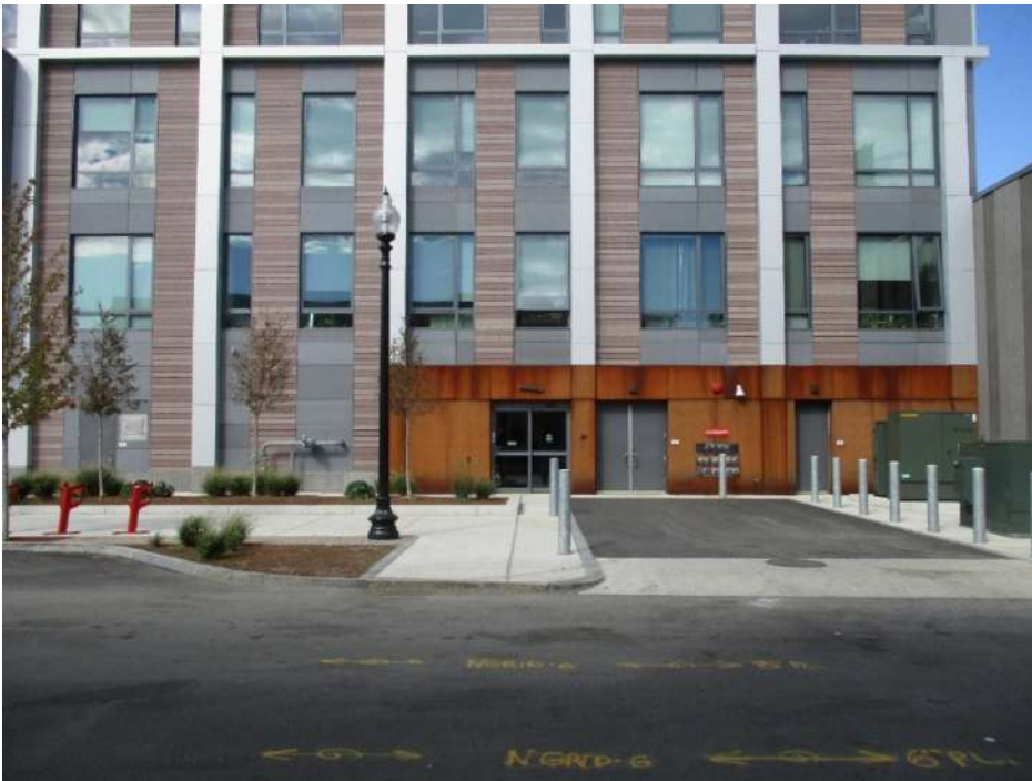
Figure 8: The ground floor elevation was elevated above the 500-year floodplain. At the new high point onsite, the design team located external transformers to save cost and space, provided fire pump access, and provided a secondary means of egress. (Source: Stantec Buildings Group.)
