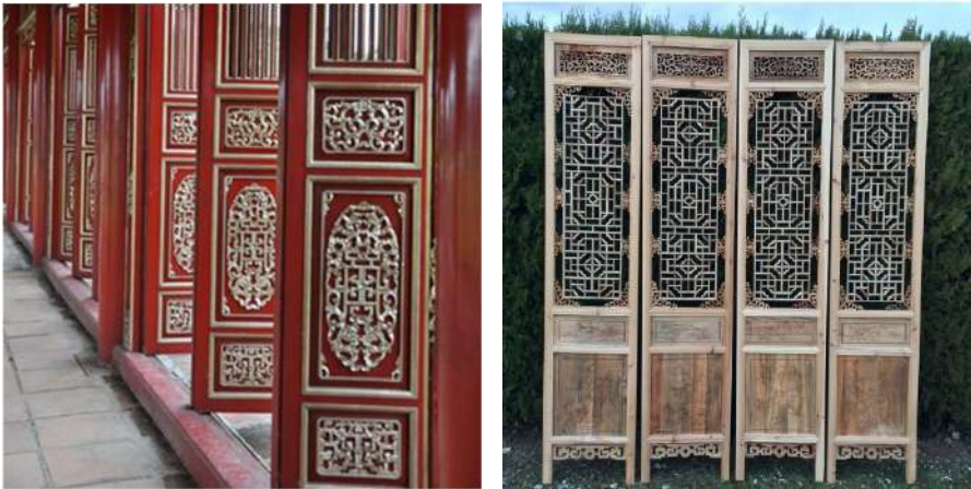
Figure 2: Left: Decorative lattice screens as means of passive ventilation and light control. Right: A movable and foldable curtain wall screen with traditional patterns. (Source: Author.)
